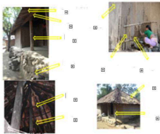
Fig 9: Arrangement of structural members in a typical Warli house:
