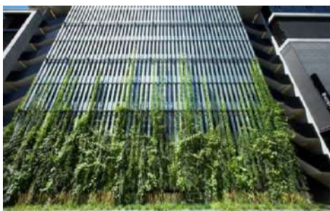
Fig 3 Green Façade Planted in to the Soil( www.selector.com )
